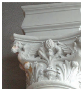
Fig. 3: Increasingly stronger in demand, especially by architects and producible by robot: building elements of complex shape, such as this capital of a classical column
